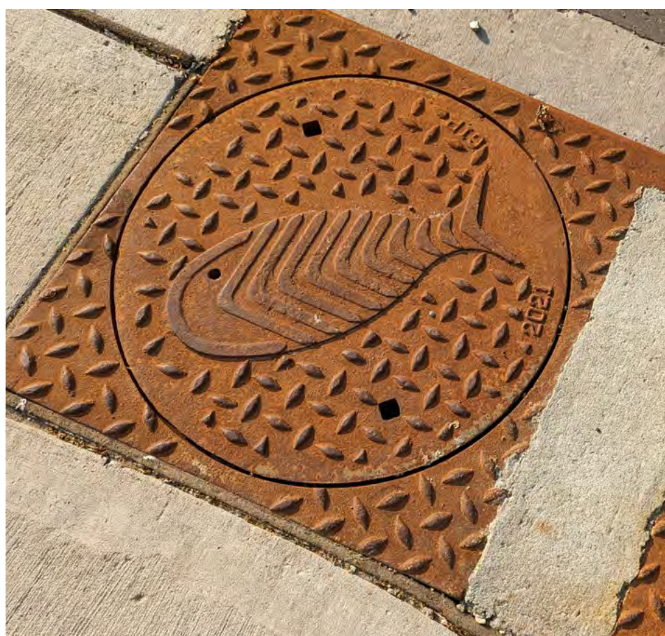
It's fishy down there? Manholes in Tillsonburg Ontario. Créditos: Stella Jurgen
