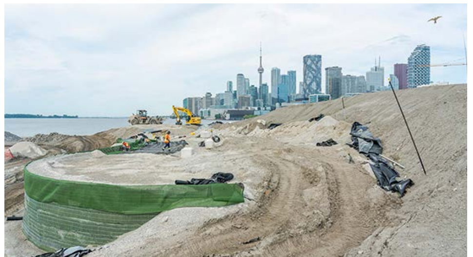
The Port Lands Flood Protection Project requires excavating, moving and placing more than 1.5 million cubic metres of soil and fill, enough to fill the Rogers Centre. Foto: WATERFRONT TORONTO/VIDINGELEVICIS/RYAN WALKER
